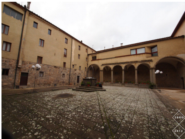
Fig. 3 - The well at the centre of the cloister of the abbey of San Salvatore offers the only access to the huge tank below
